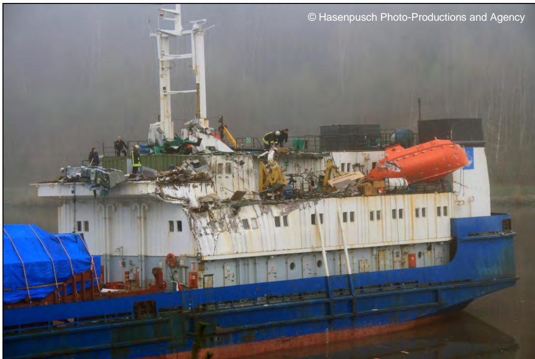
Figure 5: TYUMEN-2, damage to the superstructures and lifeboat
