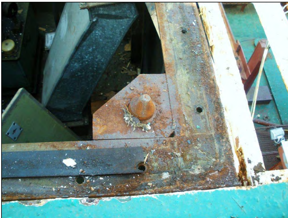
Figure 18: TYUMEN-2, installation cone at the outer corners of the foundation of the wheelhouse, irregular hole spacing of the screw connection and rubber layer
