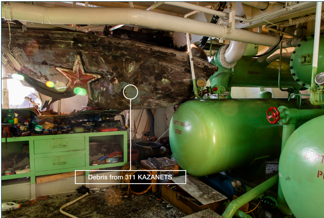
Figure 16: Debris found in ICE ROSE Source: DMAIB
