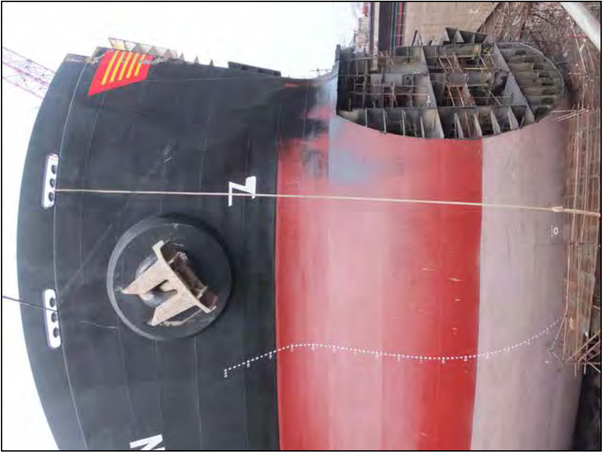
Figure 9: Chou Shan's bow under repair
