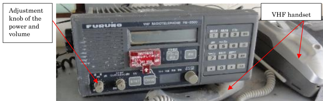
Photo 2.5-5 VHF (repatriation of after lift-up situation)
