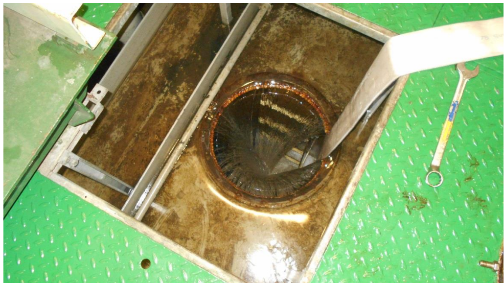
Fig. 19. By opening this man hole, in spite of the water level in the room rising, it was possible to lead the water away from the pump room. Image: Stena Line.
