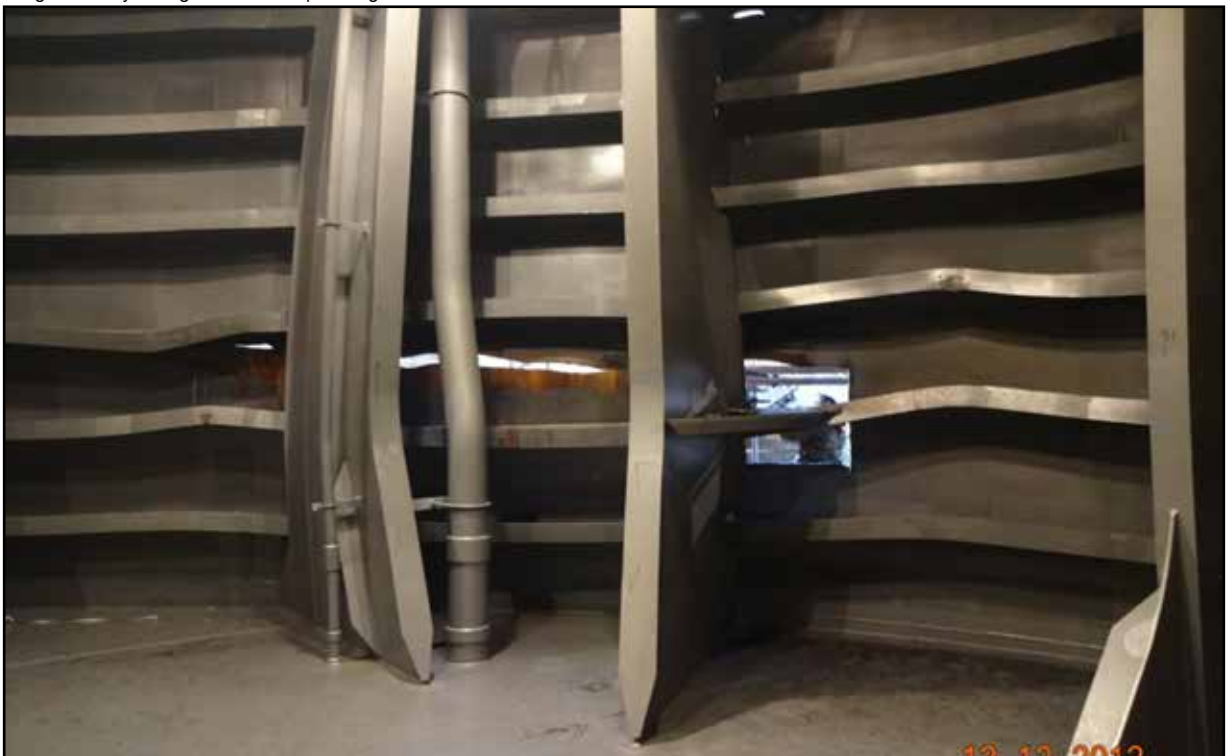
Figure 8: Damage to Darya Gayatri
