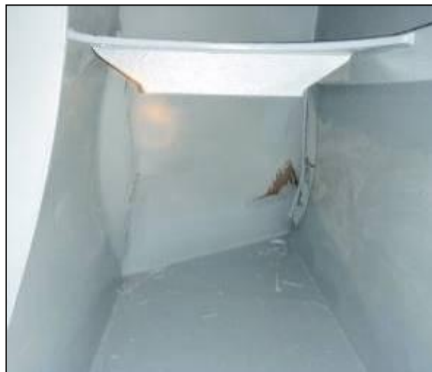
Figure 20: Stiffeners buckled and side shell indented
