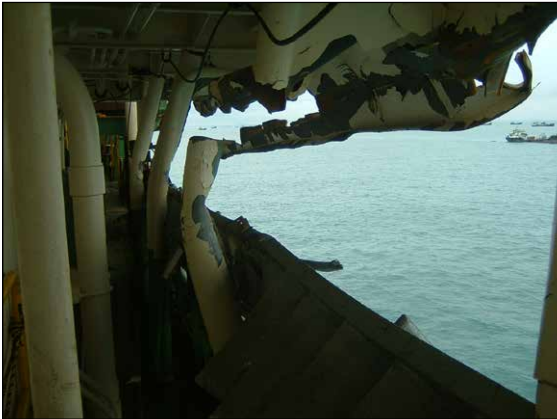
Figure 12: Damage to Hyundai Discovery 's port side accommodation section
